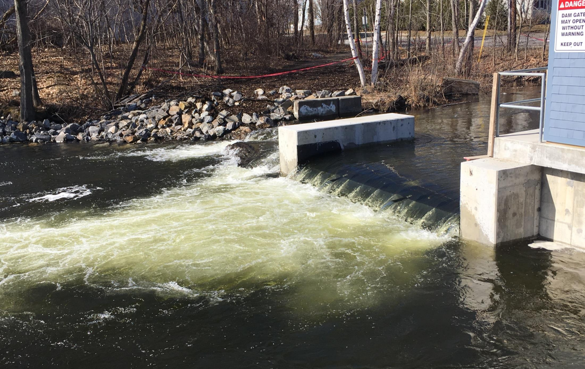
Reconstructed Maranacook Lake Dam: improved water discharge and lake level control
